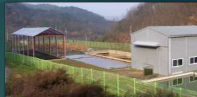
MIRECO Water Treatment Facility
