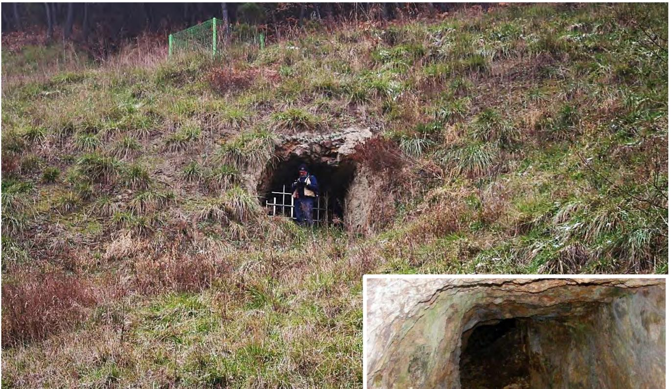
View looking north of the East Adit portal, driven along the *East Vein* for 550m. Revegetated grass cover has been effectively established. A small gate has been erected by MIRECO to bar entry to the public, but the adit remains accessible for re-entry and sampling underground. The sandstone host exhibits intense vein and fracture stockworks, argillic clay alteration and limonite staining after sulphides.
