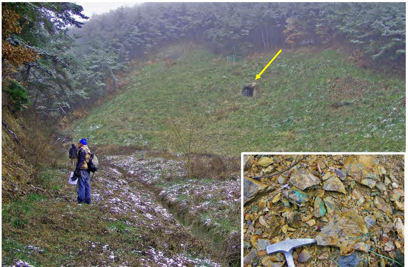
Dongil South. Outcrop of the copper mineralization (inset) of the *Central Vein* at left and the East Adit portal driven along the *East Vein* (arrow). Note the revegetated grass over the cleared, clay altered subcrop to stop erosion and concrete drain installed by MIRECO.
