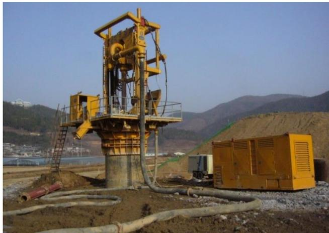
The Pile Top RCDs are manufactured in Korea and can be fitted with drill bits of 1.0-4.5m diameter. The Reverse Circulation drilling method (RCD) is used with airlift in water to lift the -2mm drill cuttings as a slurry to surface.
