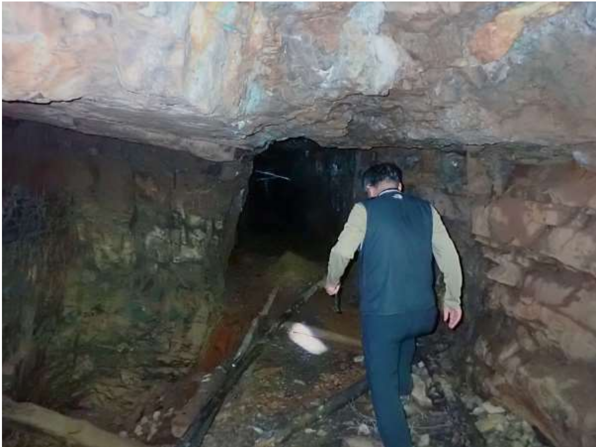
Photograph 20. Looking along strike at the steep-dipping vein breccia exposed in the adit roof at Jukdong North.
