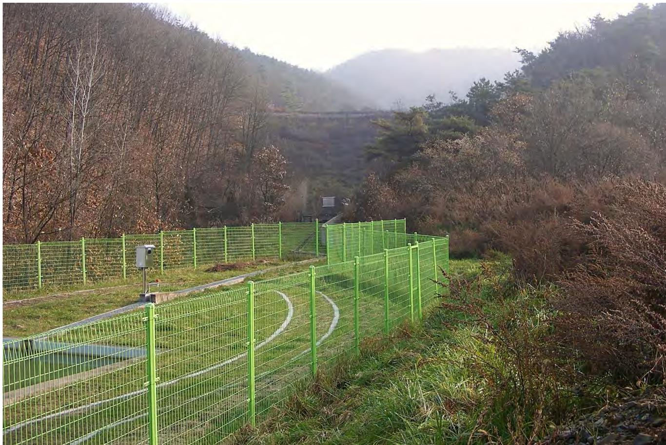
**Capped Tailings Storage Facility at Jeonheung, with a water monitoring device on the drain collecting runoff at the MIRECO metals recovery and mine water treatment plant. The mine tailings probably contain a low-grade resource that could be exploited in any future development at the project.**
