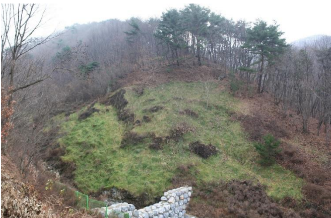
Revegetated mine workings at the Goroseoksan mine. A rockwall silt trap placed in the creek is evident in the foreground.
