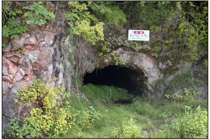
The No 2 Adit was driven along the No 1 Vein for a distance of 20m.
