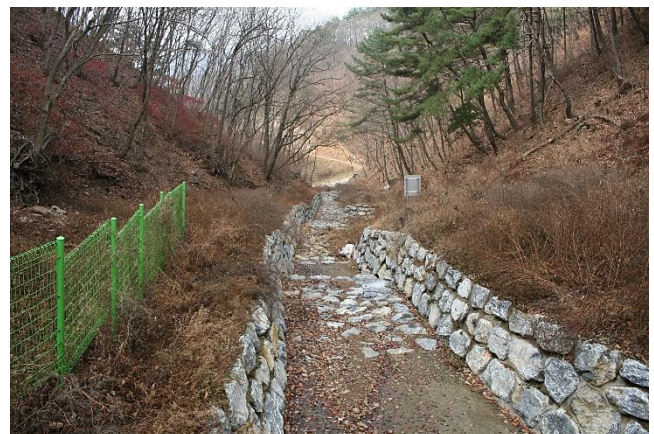
Rock retaining wall and silt trap placed in the creek draining the Goroseoksan mine workings.
